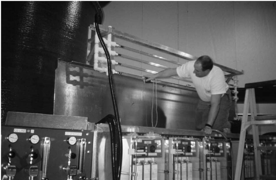
Fig. 7. Quartz sleeves are cleaned on an open channel UV system (with low pressure/low intensity bulbs) at the Freshwater Institute.
