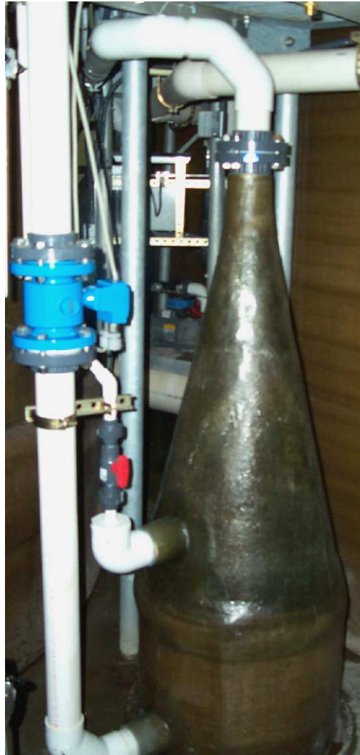
Fig. 4. A down flow bubble contactor was used to remove off-gas from the side-stream flow before it entered the UV irradiation chamber.
