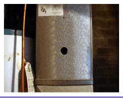
4. Place the UV tube bracket plate over the hole with the black plastic tube mount in the center of the hole with the stickers on the outside as shown. Mark the 4 holes in the corners, Remove the mounting plate and pre drill the 4 holes with a 3/32" or smaller drill bit.
