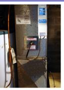
7. Plug the UV cable from the control box into the UV tube. Plug the DC plug from the desktop adapter into the control box. Make sure the power switch is turned off and then plug the desktop adapter into the wall receptacle.
