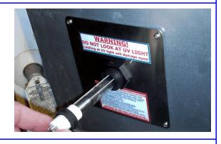
3. In a normal situation the tube will just need to have the dust removed. This can be done using a dusting cloth such as a Swiffer® duster or Swiffer® cloth.
