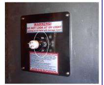
2. Remove the rube by carefully sliding it out.
