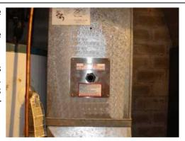
4. Place the provided ozone resistant Norprene seal ring in the middle of the ceramic socket on the tube, slide the tube into the tube mount, being careful not to push it past the Norprene seal. Install the plastic retaining nut and tighten very tight.
