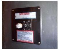
5. Next place the control box in the desired place and mark the 4 mounting holes. Make sure the control box is being mounted in a location that will allow the 2 ft or 10 ft cable to reach the UV tube. Pre drill the 4 holes with a 3/32" or smaller drill bit. Place the box back in place and install the 4 provided stainless steel screws.
