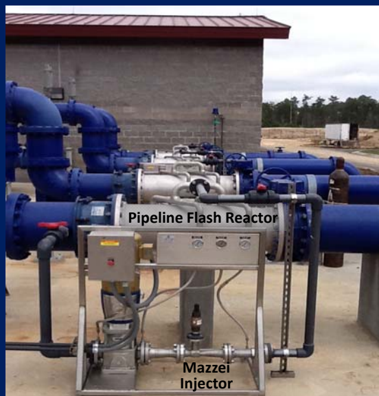
Waste Water Effluent Aeration Hancock County, MS, USA
